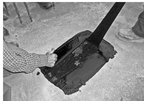
Figure Y – Cohesive failure (pass)
